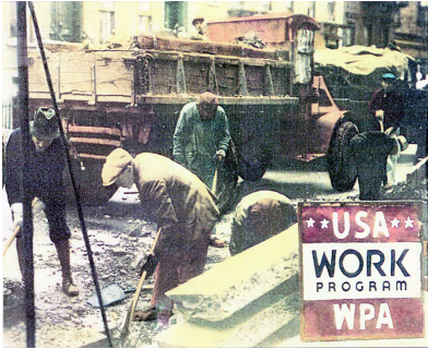
Works Progress Administration (WPA)
